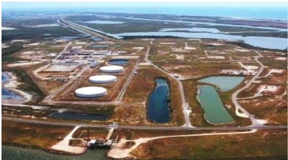
An aerial view of the Bryan Mound storage site of the Strategic Petroleum Reserve Photo: U.S. Department of Energy
